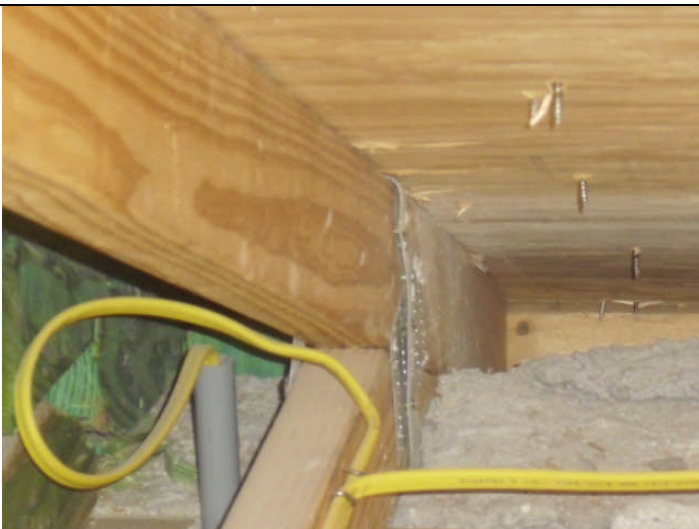
Roof to wall attachment
