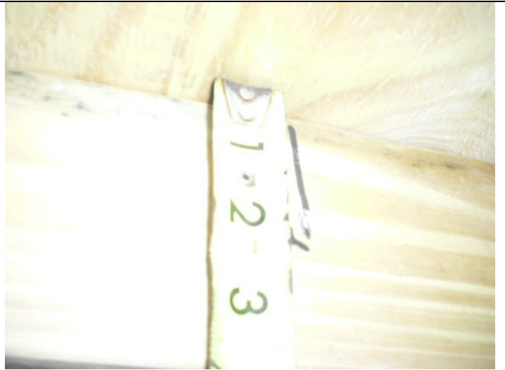
Roof deck attachment
