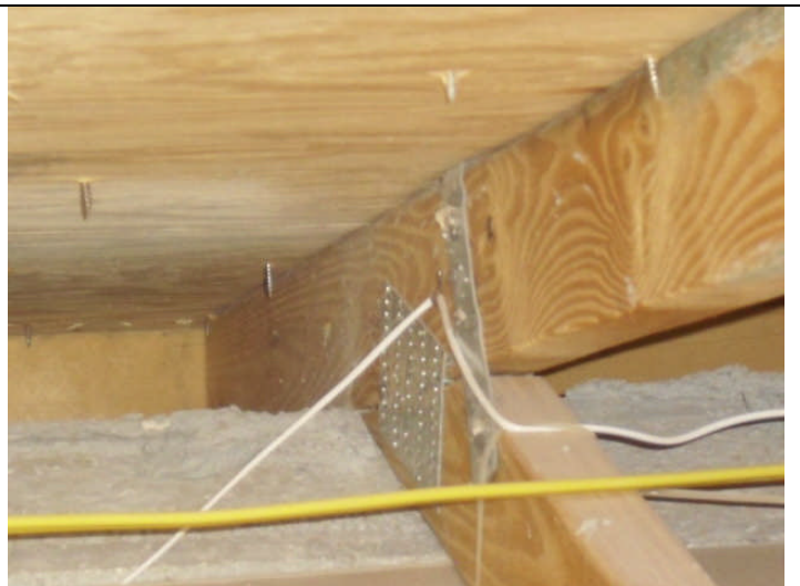
Roof to wall attachment
